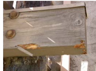
Photo: 26 - Drywood termite damage, Incisitermes , family Kalotermitidae Photo: Dr. Vernard R. Lewis
